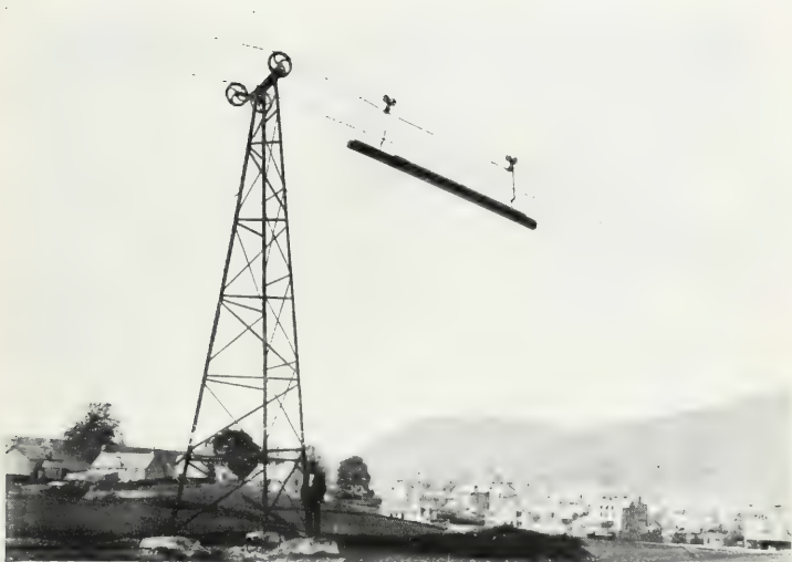
FIG. 61. AERIAL ROPEWAY: A TRESTLE AND CARRIAGE.
